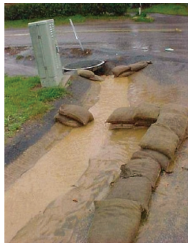
Figure 5. Make sure storm drain inlets are protected.
